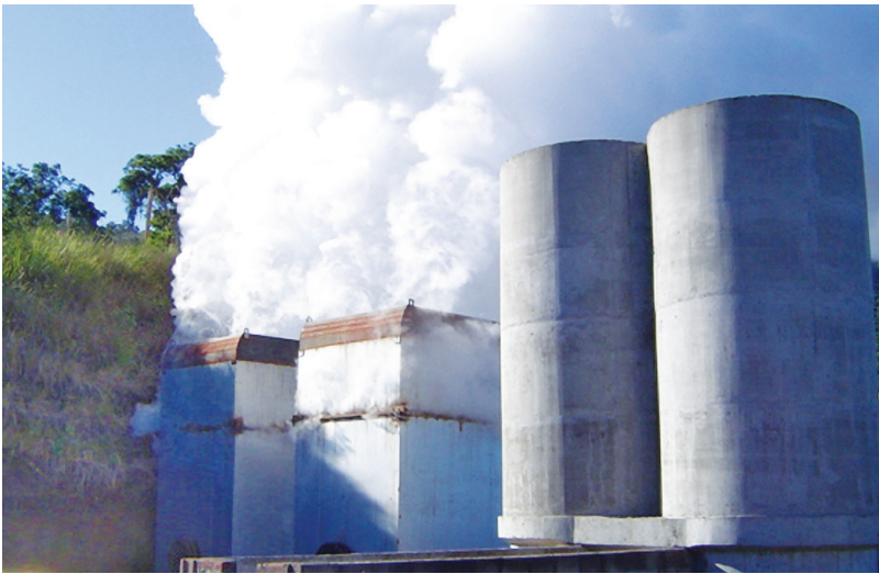
Fig. 3. Rock mufflers in El Salvador (Courtesy LaGeo).
