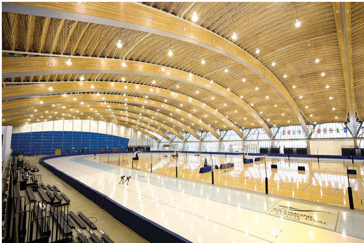
Fig. 7. Main Hall and rink with skaters (Photo by Stephanie Tracey www.photographywest.ca Courtesy Wood WORKS! BC).
